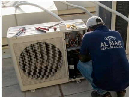
Sheikh Khalifa Hospital, Ras Al Khaimah
